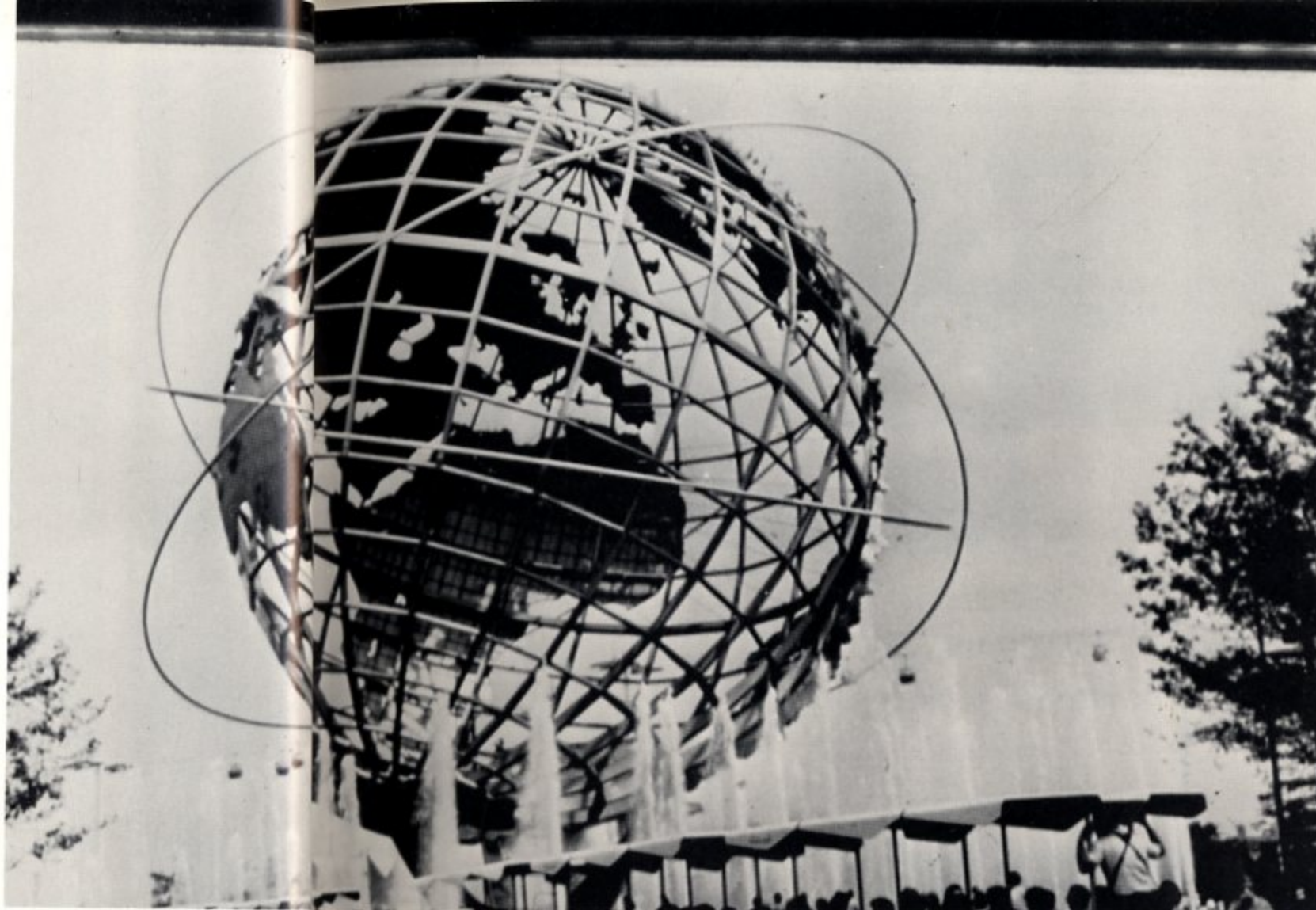
The Unisphere, a structural steel model of the world is 140 feet high. Land masses are supported by an open grid framework of latitudes and longitudes. Floating around it are the ringed orbits of man made satellites. These pay tribute to man's probing of outer space.
