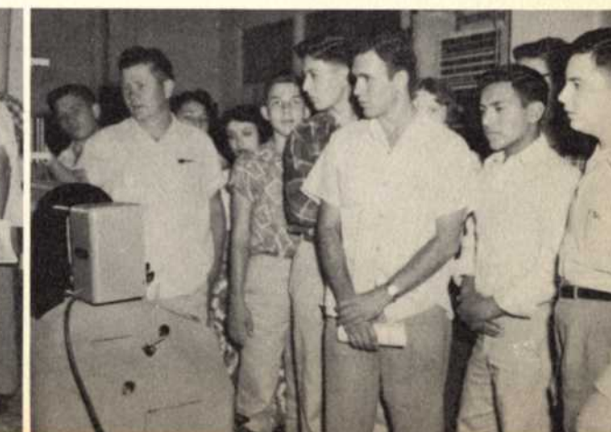
Mr. Henderson shows how line network broadcasts and teletype messages are received. All the club members were surprised to learn thirteen or more calls come in on one channel or wire.
