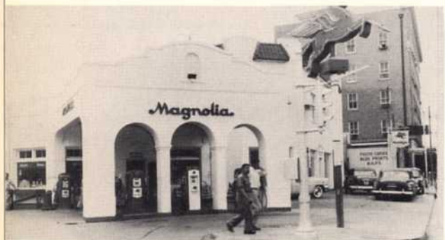
SPENCE SERVICE STATION 1210 Matamoros Laredo, Texas
