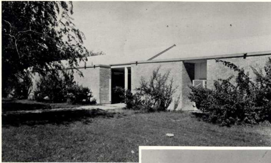
The bougainvillea blooms frame the home-making cottage which now sports air conditioning.
