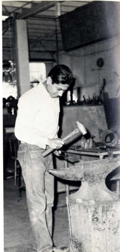
Dionicio Solis is forging a chisel.
