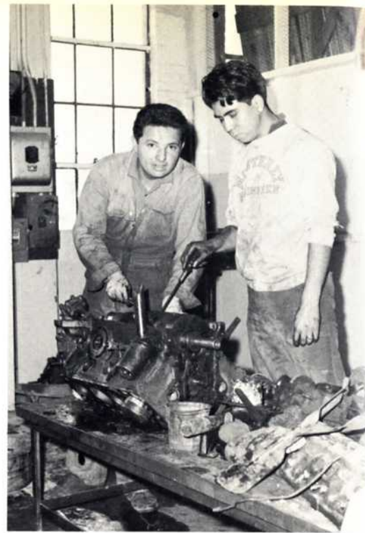
Mr. Cortez explains to Jose Coronado how to remove the camshaft on 6 cylinder engine to install camshaft bushings.
