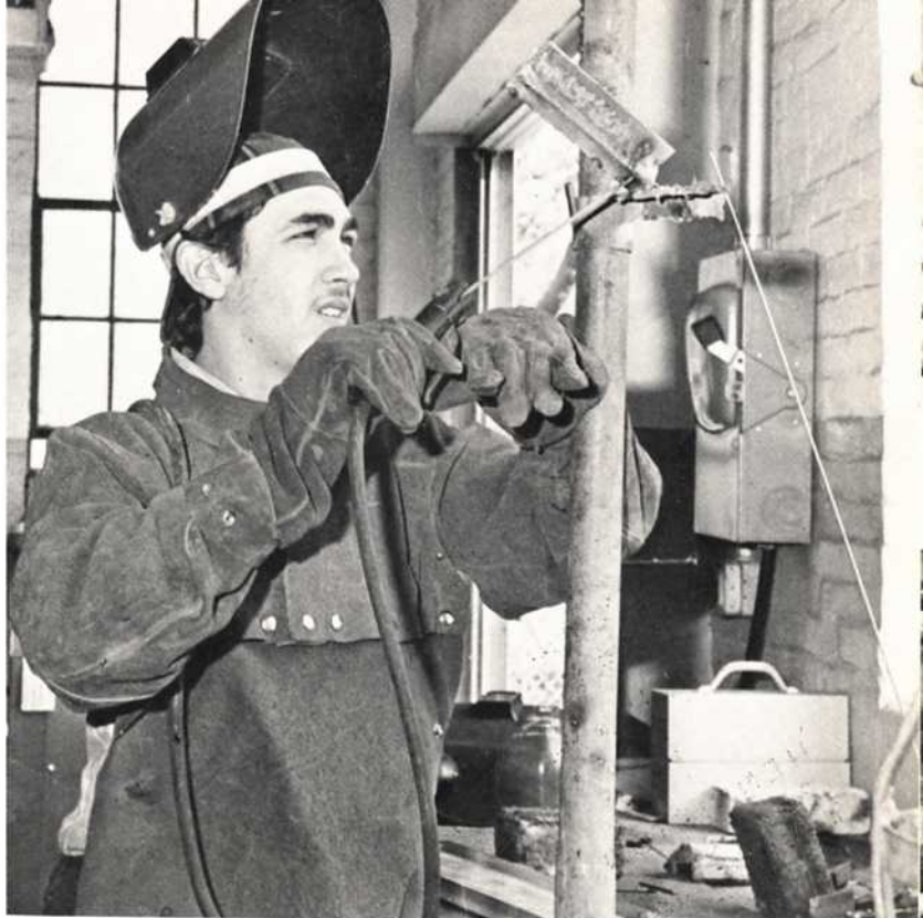
Heberto Rendon working on Low Hydrogen Arc Welding Overhead.
